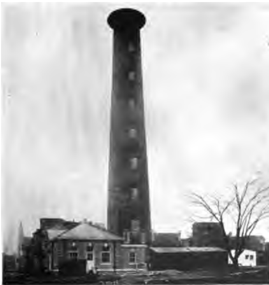
SPARKS' SHOT TOWER, FRONT AND CARPENTER STREETS (See page 99)
